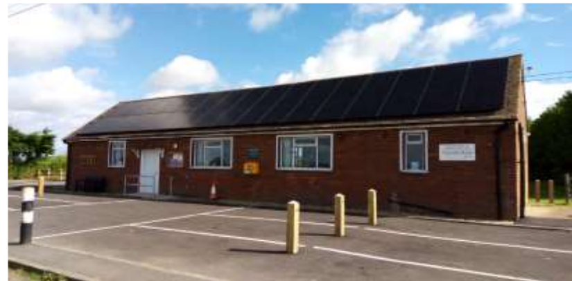
Image 2: Solar PV was installed on the roof of Graveney and Goodnestone village hall through the Community Infrastructure Grants.
